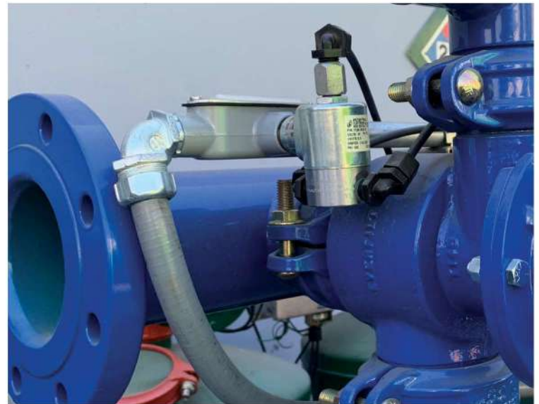
INDUSTRIAL TYPE SOLENOID INSTALL: ( M, A, I )
