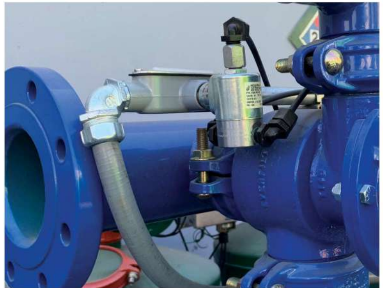
INDUSTRIAL TYPE SOLENOID INSTALL: ( M, A, I )
